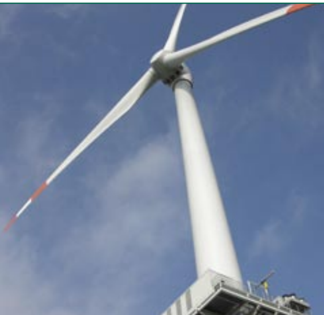
External view of the 120m high Multibrid M5000 at Bremerhaven
